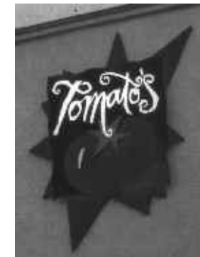
Layered aluminum shapes. Routed copy backed with acrylic. Internally illuminated with fluorescent lamps.
