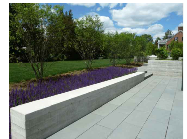
Seatwall Cast In Place Concrete
