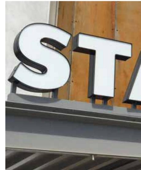
Upright Mounted Pan Channel Letter w/ Raceway Internally Illuminated
